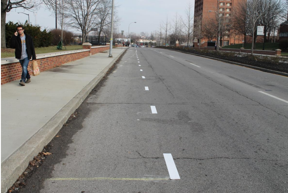
Figure 50: The Extension Line of the Third Survey of the Newly-Developed Countermeasure for Bicyclist Safety-Part 1
